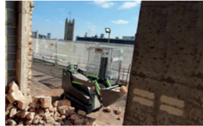
City construction / Demolition / Landscaping
