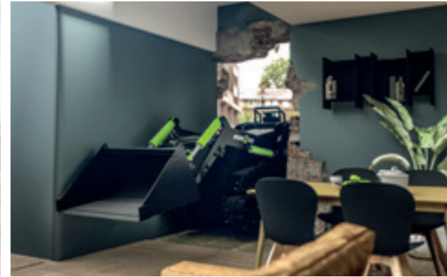
Interior construction / Demolition
